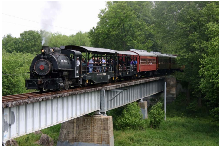
Above: Jeddo Coal Company 85 is depicted crossing the Monocacy River. 22. May, 2021. Image: Alex Mayes.
