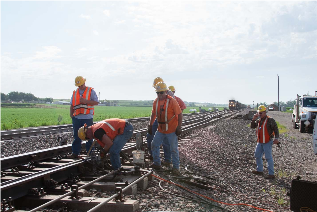
Above: A westbound Union Pacific freight train approaches Union Pacific track and signal staff inspecting a turnout at Control Point Gerry (just west of Hanover), Kansas. July 2, 2008, 07:23.
